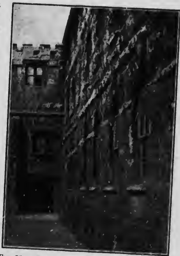
FIG. 37. — Weathering of limestone in the wall of an old building: Trinity College, Oxford, England.
